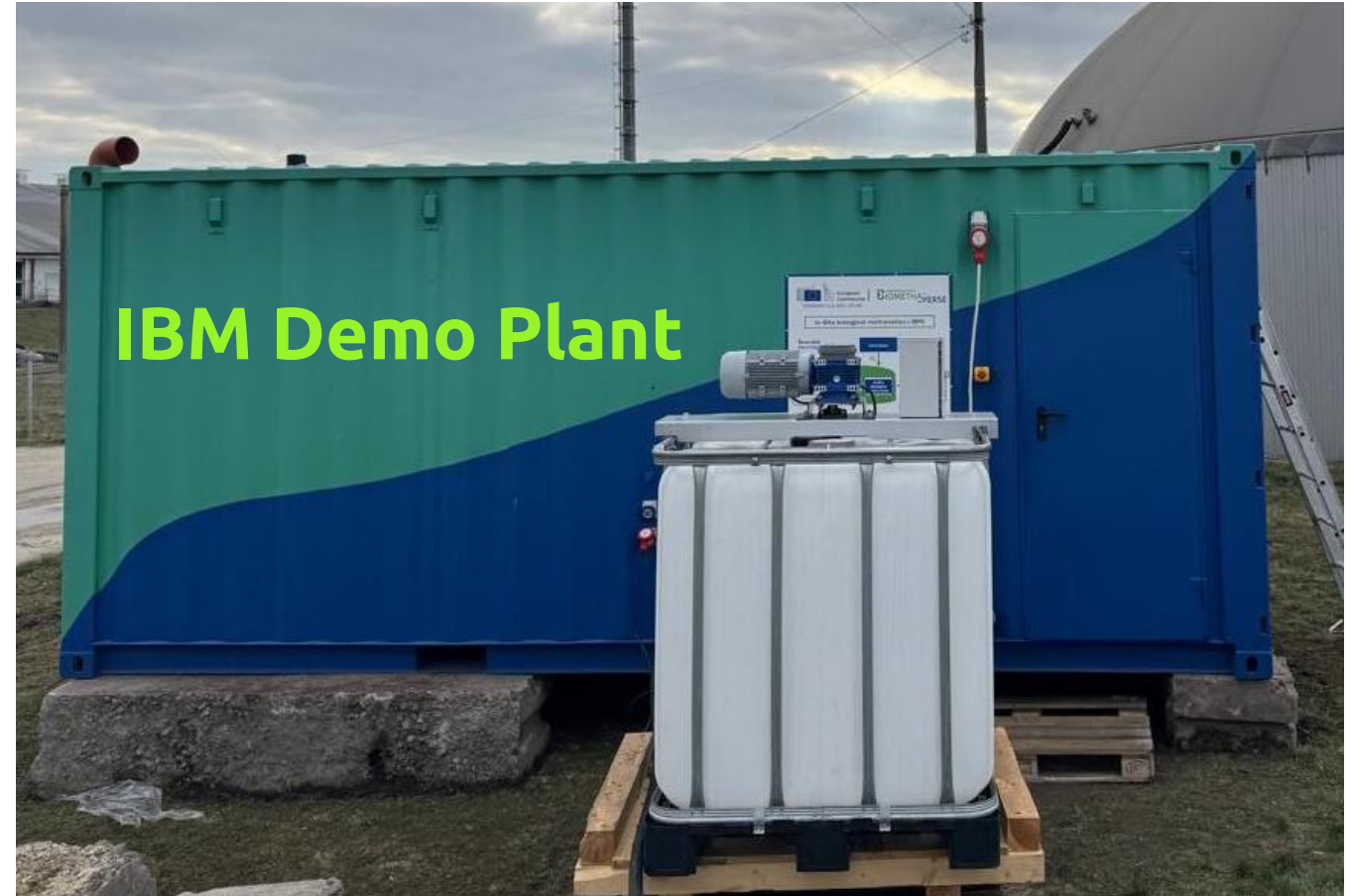
Containerized In situ Demo Plant Ukraine
