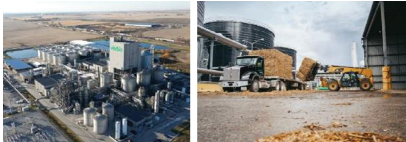
Fig. 9.4 – VERBIO Nevada Biorefinery biomethane plant
