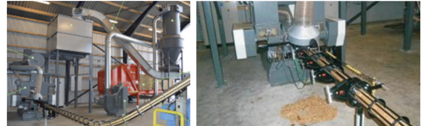
Fig. 9.2 – Straw briquette feeding line
