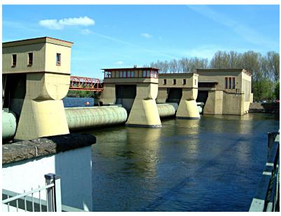
The 3.3 MW run-of-river HPP Hengstey between Herdecke and Hagen (Germany). The plant operates with three Kaplan turbines and generates 11 million kWh/year. Source: Wikimedia Commons CC BY-SA 3.0
