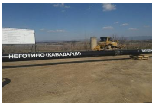
Picture 7. Construction of Lot2
