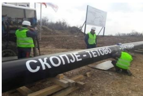
Picture 6. Construction of Lot5
