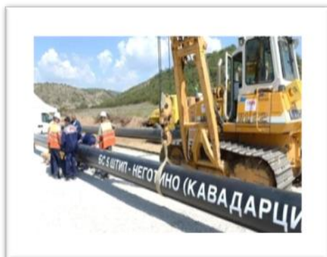
Picture 5. Construction of Lot1
