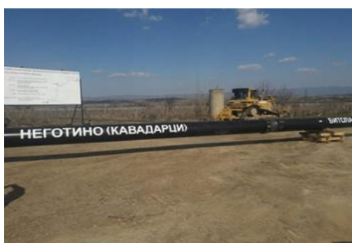
Picture 7. Construction of Lot2
