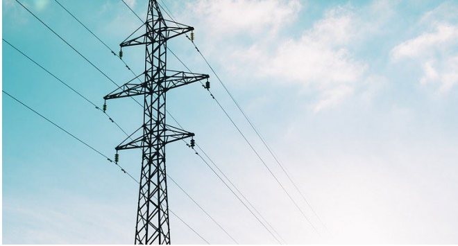
Construction of 84 km of double-circuit 400 kV overhead transmission line from Bajina Bašta to the Bosnia and Herzegovina and Montenegro borders, the last section of the Trans-Balkan Electricity Corridor in Serbia
