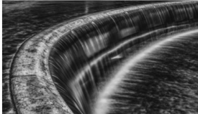
Electro-mechanical rehabilitation of six large hydropower plants with a total installed capacity of 443 MW in North Macedonia
