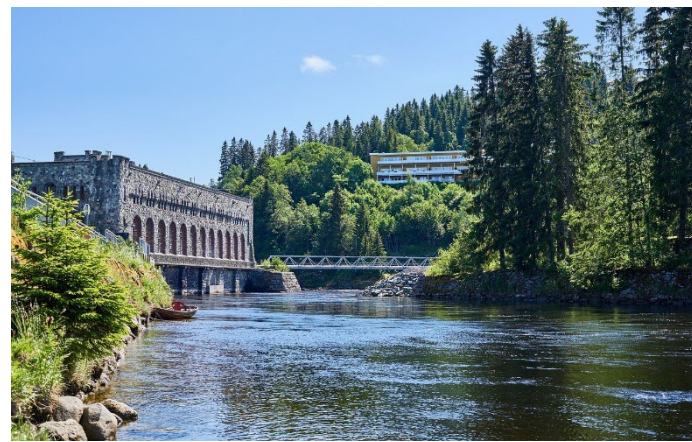
Electro- and hydromechanical rehabilitation of 220 MW Čapljina hydropower plant in Bosnia and Herzegovina
