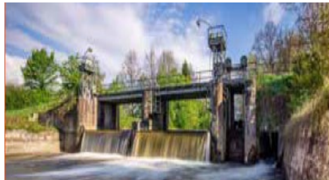
Electro- and hydromechanical rehabilitation of 136 MW Vlasina hydropower system in Serbia
