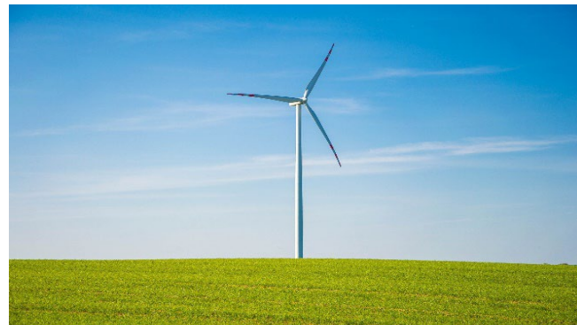
Installation of a 66 MW wind farm on the site of depleted open-cast mines in Kostolac, Serbia
