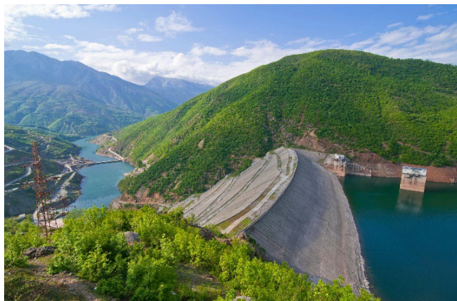
Electro-mechanical rehabilitation of 500 MW Fierza hydropower plant in Albania
