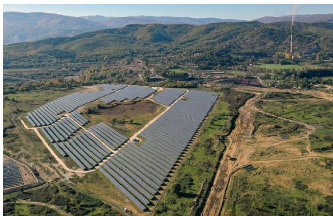
A 10 MW solar power plant was installed on the site of the exhausted coal mine in Oslomej, North Macedonia (completed in 2022)
