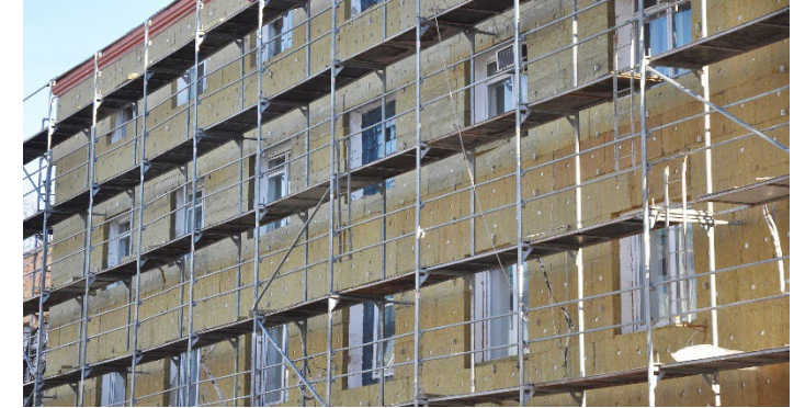
Renovation of 17 healthcare facilities in North Macedonia
