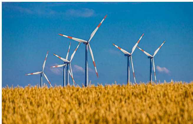
Installation of a 132 MW wind farm in Poklečani in the West Herzegovina Canton
