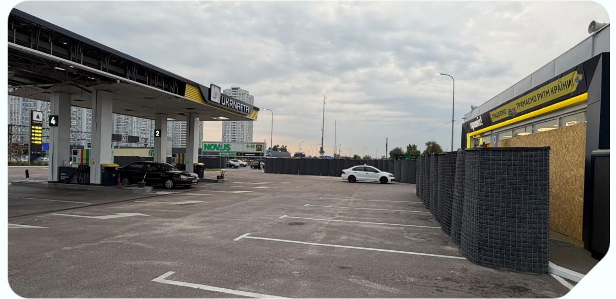
Recovery: clearing debris, temporary facade protection and preparations to reopen
