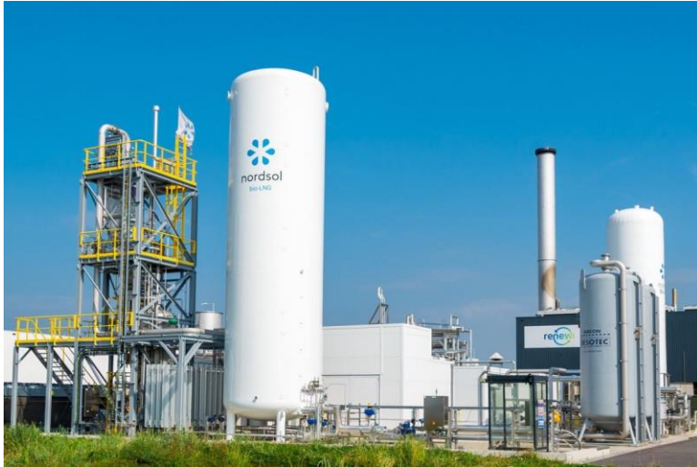
bioLNG liquefaction plant in Cologne, Germany under construction – capacity 100kt bioLNG per year
