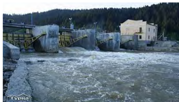
Figure 27 Small HPP in Turka
